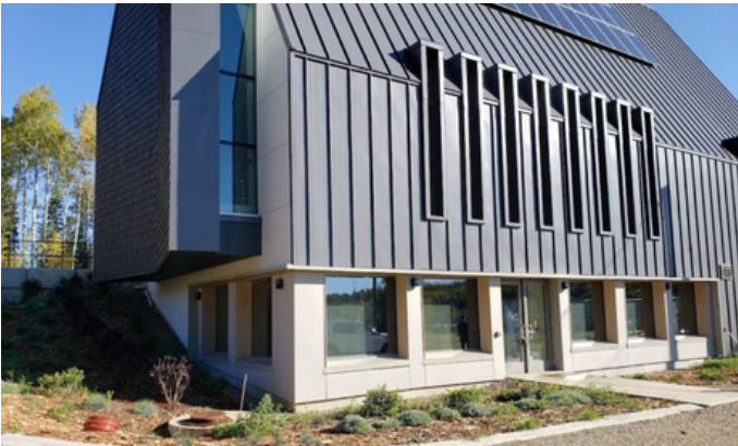
The building's location and direction help maximize winter light, minimize heat loss, and collect solar power on the rooftop.
