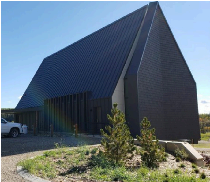
The building won three Architecture and Passive House awards.
