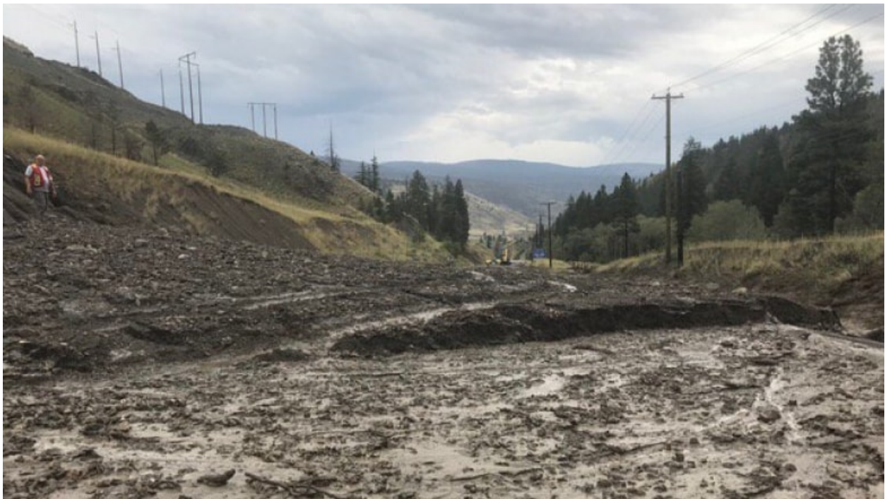
Figure 1-5. Debris flow blocking Highway 97 south of Clinton, BC on July 31, 2018 (MOTI, 2018). This area was burned in 2017 by the Elephant Hill Wildfire.
