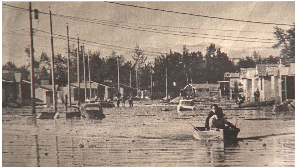
Figure B-7. Flood event of June 2, 1972 when dikes along the North Thompson River failed and sent flood water into the Oak Dale Trailer Park in Westsyde, near Kamloops BC. (CFJC Today, June 2, 2017).
