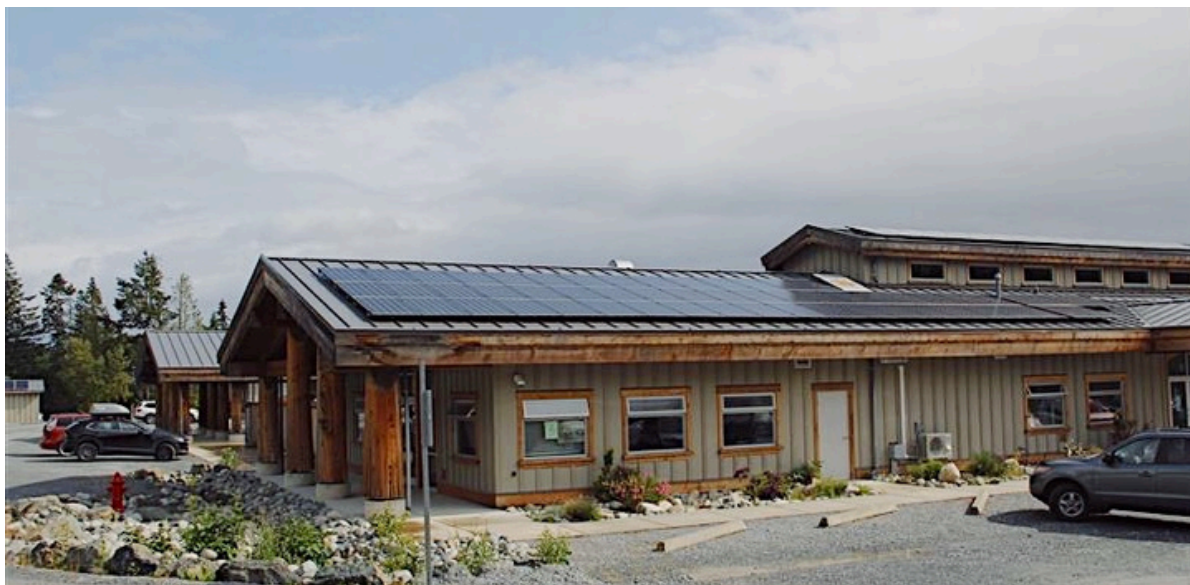
Malahat's community building with roof solar installation | Photo credit: Sybil Zhang
