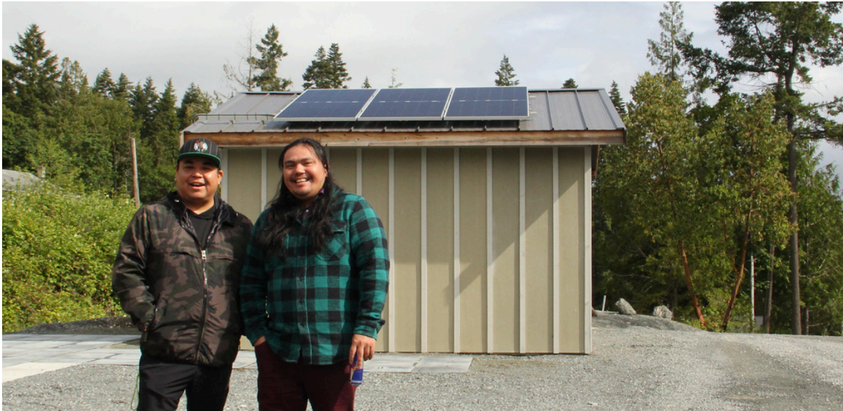
Malahat Community Energy Champion George Harry (left) and EPIC Program Lead, Kevin Good (right) in front of a storage shed with roof solar. The community is doing extensive work on solar power, including for its main administrative building, and is advancing work on other renewable energy sources. | Photo credit: Sybil Zhang
